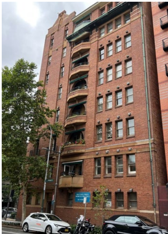
'Kingsclere' to the east - opposite side of Macleay Street
